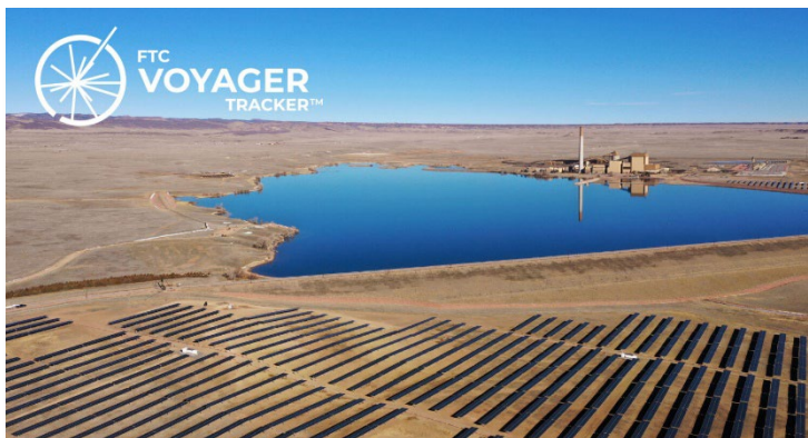
EPC Contractor Colorado – 29 MW
